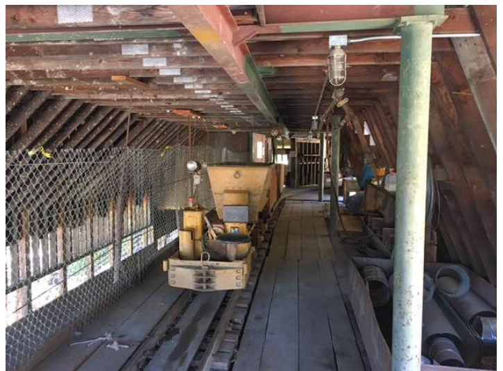
Electric Trammer & Ore Cars Inside Mill Building
