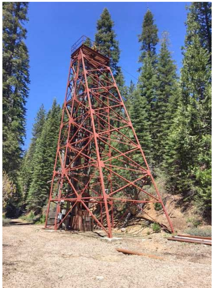
Lawry Shaft Headframe
